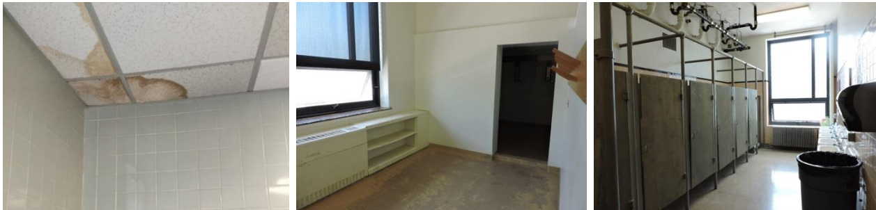
Photograph 2: Locker and Restroom Facilities
